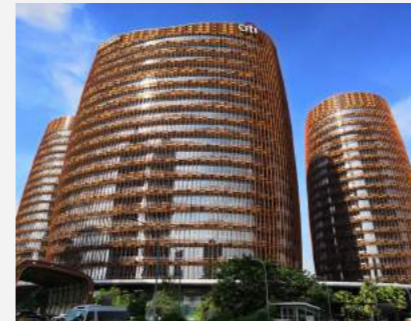
South Quarter, office
